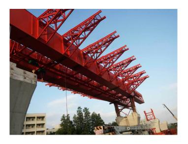
900T Overhead Movable Scaffolding System Bridge Construction
