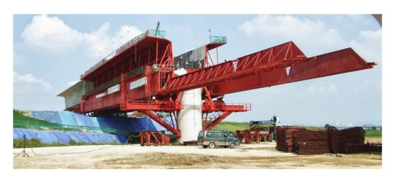
MSS is very useful when Segmental construction or other cast-in-place methods are not economical or are not possible.
