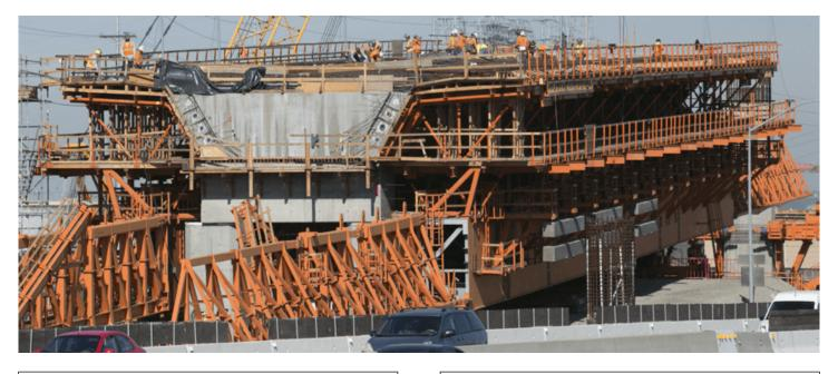
Underslung MSS has all the advantages similar to its overhead model, except that it gives additional users friendly feature by providing a clear space above the formwork.
