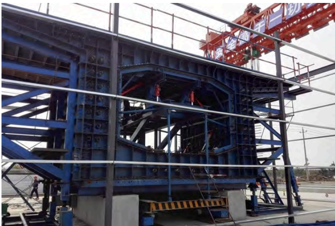
1 Set Precast Segment Moulds for the Segmental Bridge Construction
