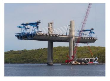
The 120 Ton 65 M Segment Lift can be optimally used in a balanced cantilever structure in which pre-casting can be carried out and the segment can be transported below the span.
