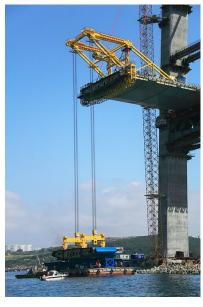
Segment Lifter is mainly divided into fixed deck crane, luffing deck crane and tower type deck crane and its derivatives products "shore crane"
